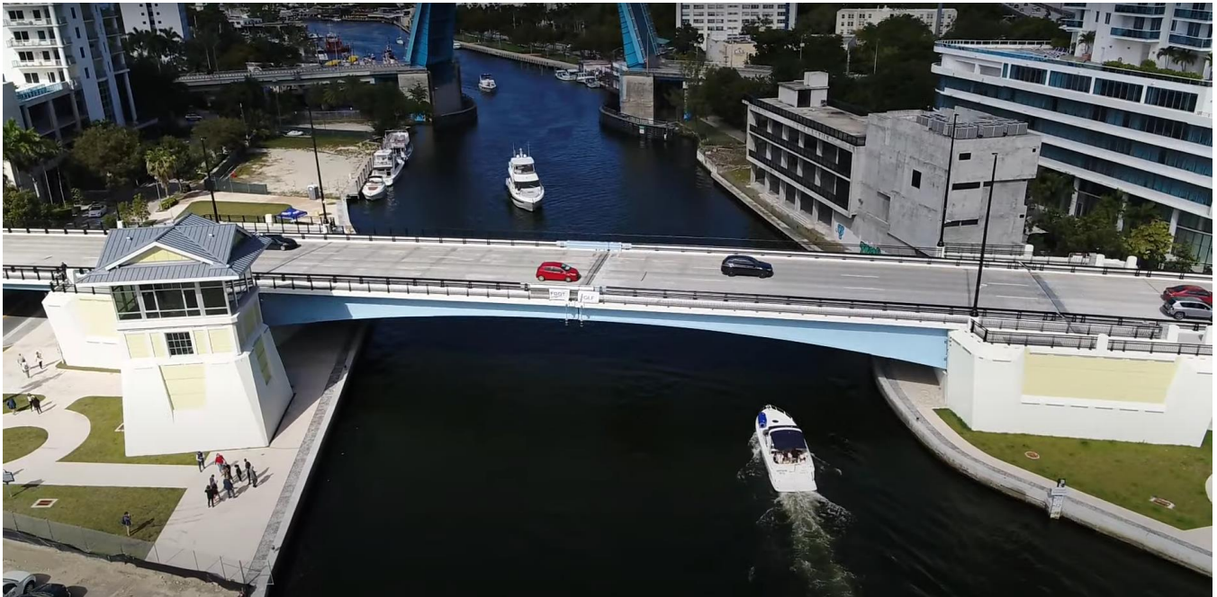
First Street Bridge
