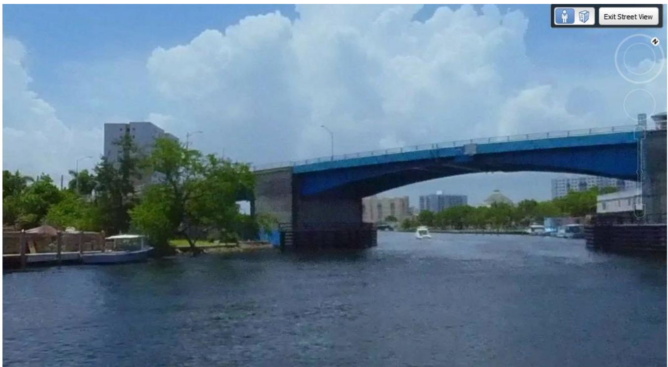
Flagler Bridge and New Park Area
